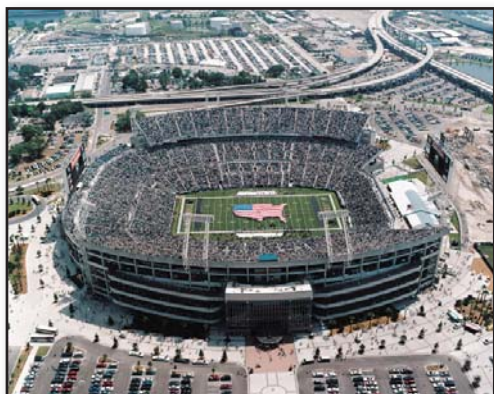
EverBank Field Renovation
