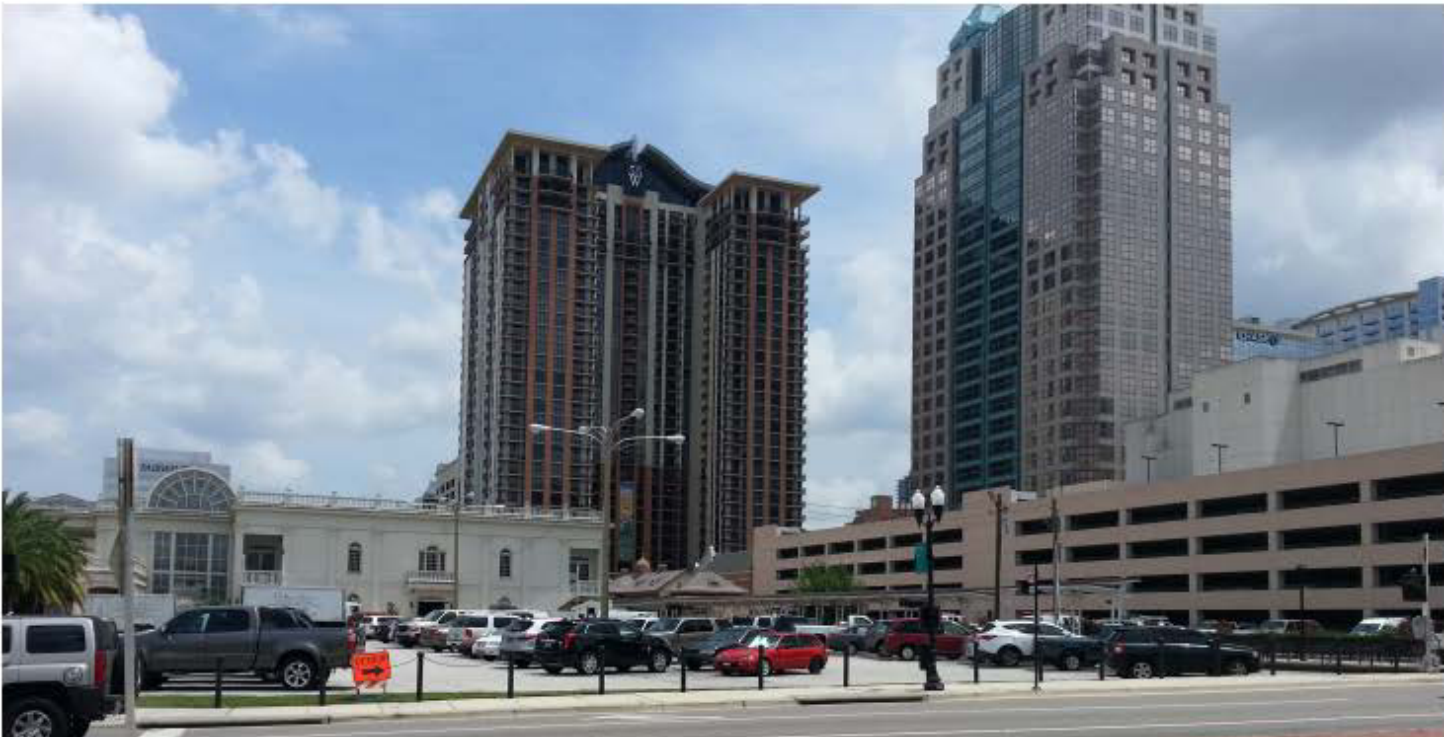
Photo #1: Google Image – Site facing Due North
