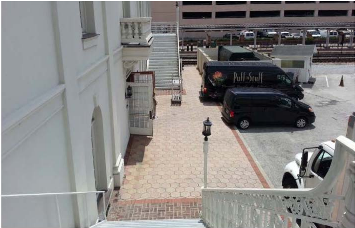
Site Photo #7: Photograph Northwest Corner Facing East
